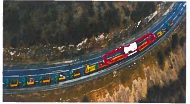
ASKI SİSTEM (GIRDER BRIDGE)
